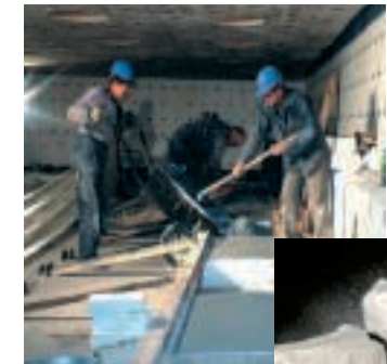
Pusher furnace with castable lining for the steel industry
