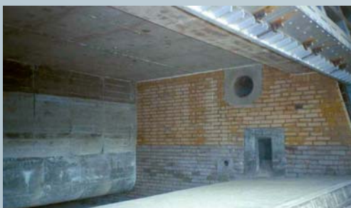
Double chamber melting furnace
