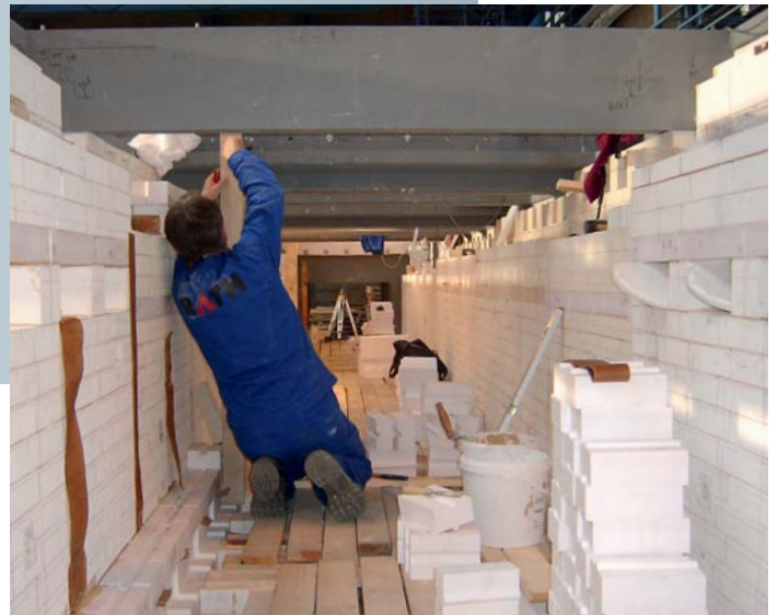
Assembly of a pusher-type furnace
