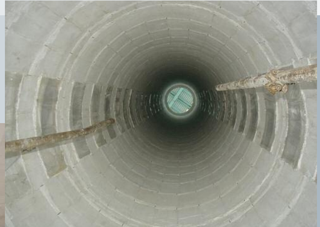
Shaft furnace with module lining
