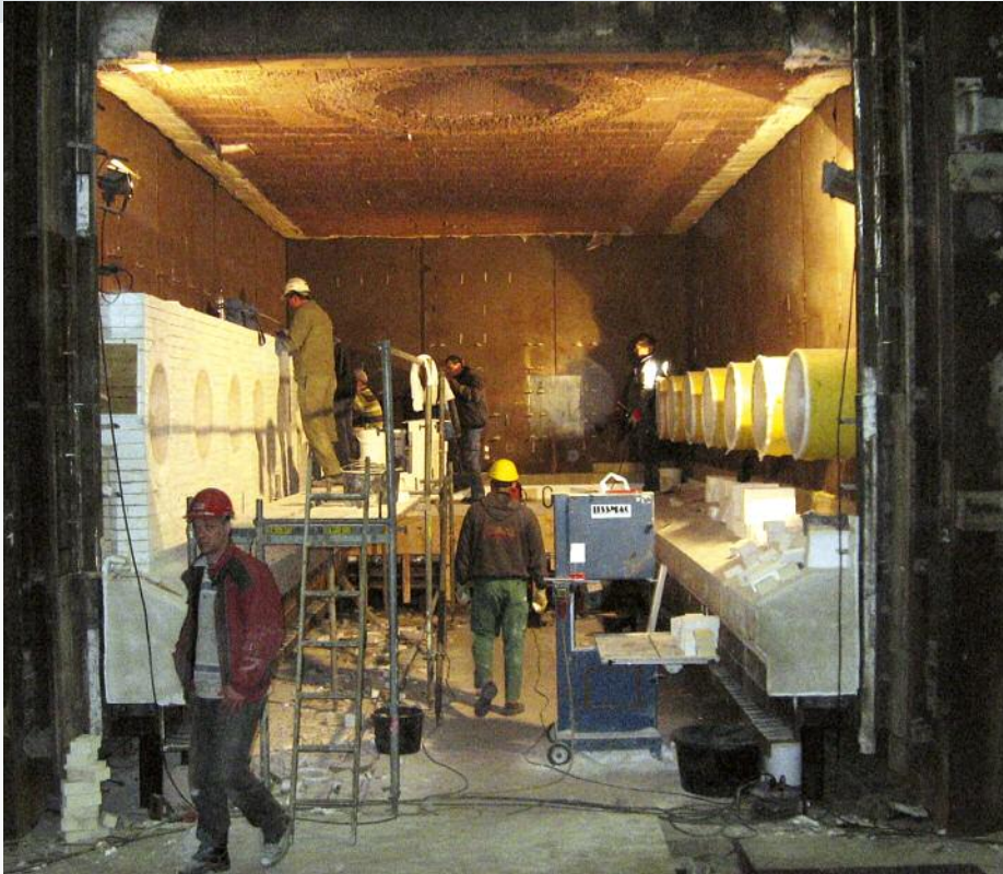
Assembly of an insulating fire brick lining
