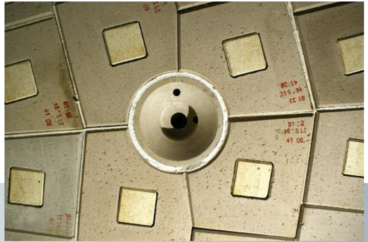
Ceiling parts of pre-cast blocks
