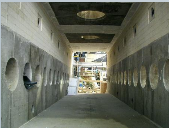
Roller furnace with new energetic optimized lining
