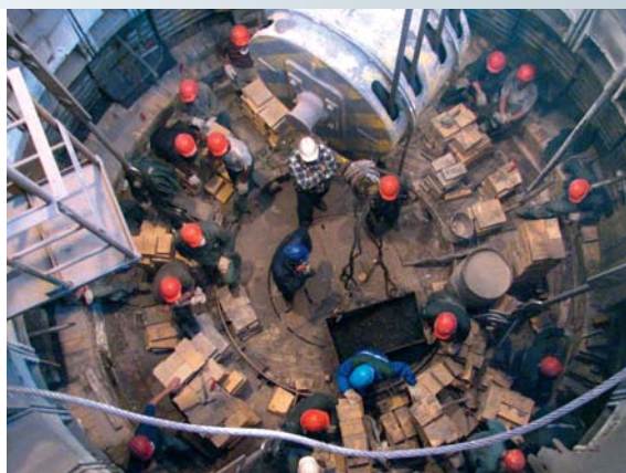
Blast furnace relining
