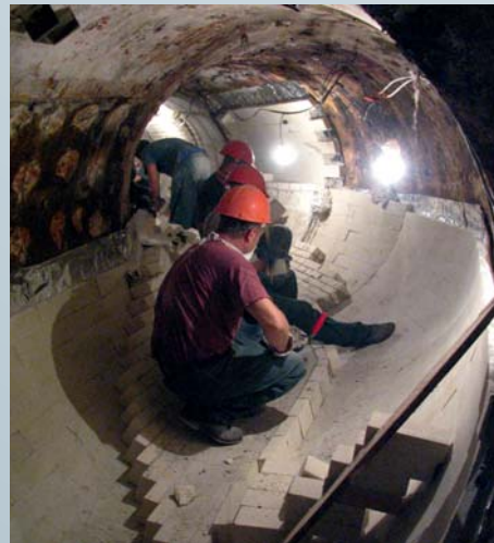
New lining of a hot blast duct
