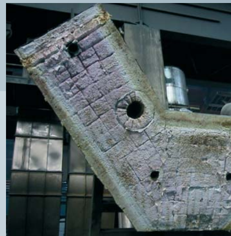
Roof of a tundish
